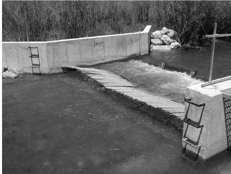
Figure 2. Floating resistance board weir in Pine Creek, Idaho used to divert upstream migrating trout into a collections box (edge of picture in foreground) for phenotypic sorting.
