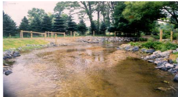
Figure 3. This after picture shows streambank fencing excluding cattle from the stream, stabilized stream banks and improved in-stream habitat. This shot was taken immediately after the restoration.
