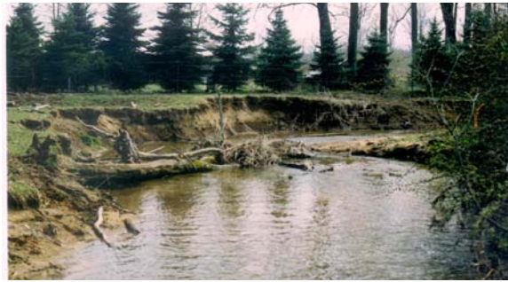
Figure 2. Severely eroded stream banks at a location in between stations 0201 and 0202. Notice pine trees in background for reference.
